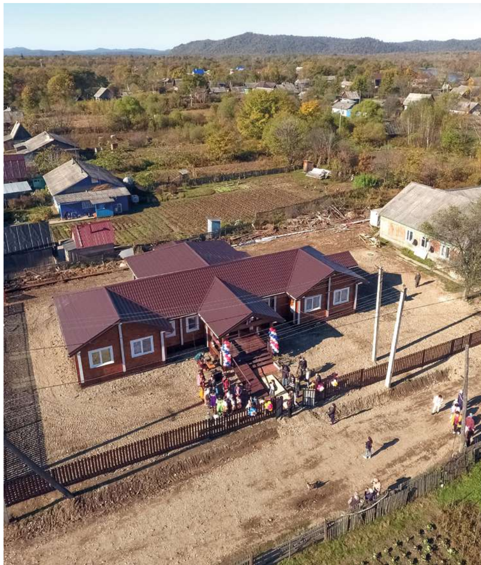
The hospital and the apartment for the doctor. The locals and the national park staff used to travel 140 km to Luchegorsk to get medical aid. Primorsky Krai administration equipped the medical rooms.
