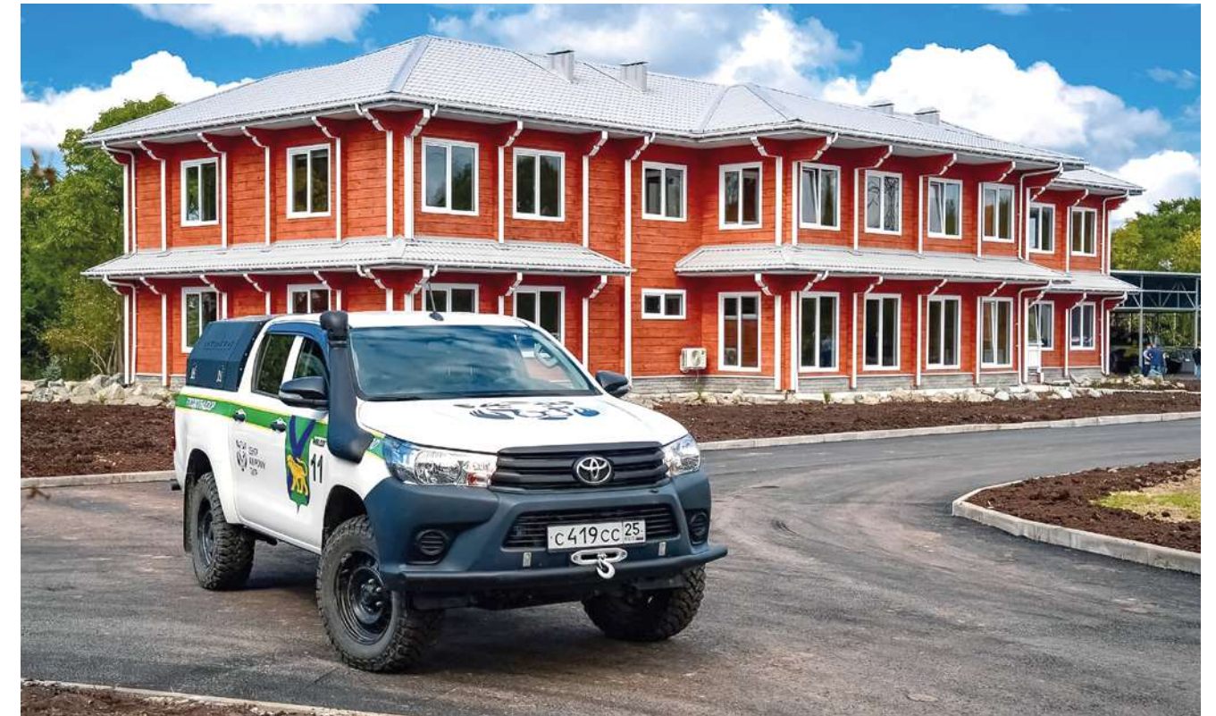
Administrative complex of the Primorsky Krai okhotnadzor
