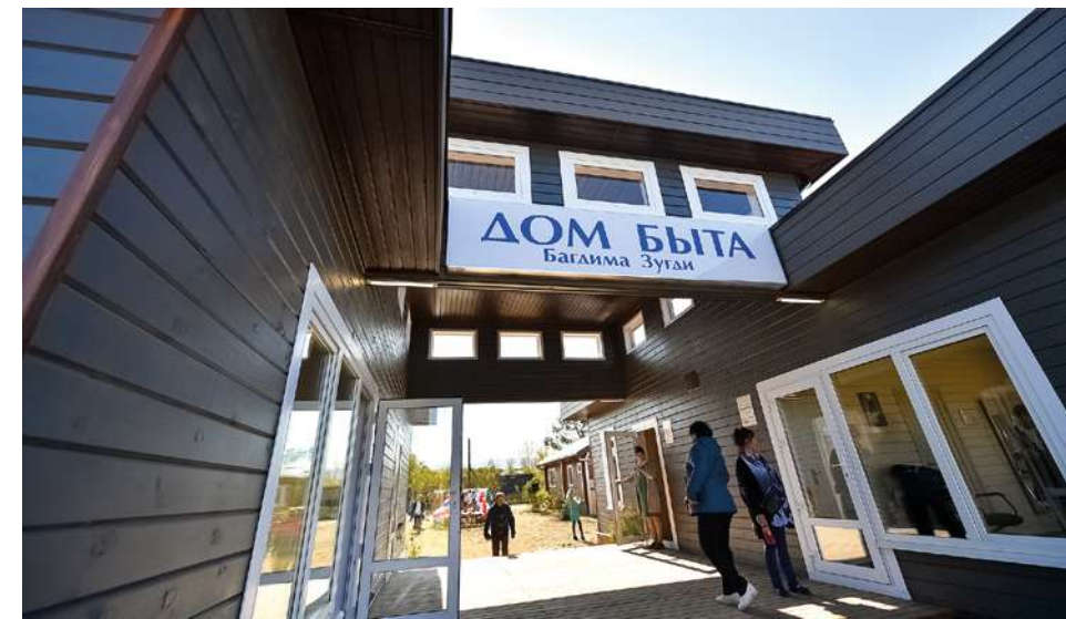
Consumer services center. The building's area is 200 m2. It hosts a beauty studio, a laundry, a food and a household store et al.
